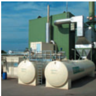
as heat exchanger in a tank
